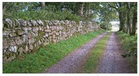
Dykes and trees don't go well together. What happens of course is the trees, if they're close to the dyke, the roots go underneath the stonework and it's not them that does the damage, it's the wind blowing the tree and the whole ground gets to it, gently shaking up and down and you lose a wall. And that's really all you need, hammer, some string and
