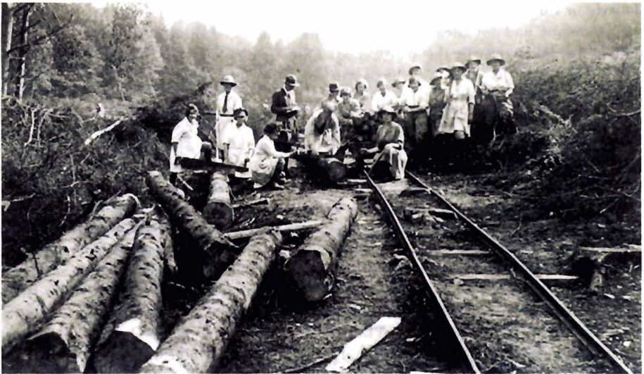
A commercial postcard of a typical short handworked temporary timber railway of 3ft gauge, somewhere in the Scottish Highlands.
