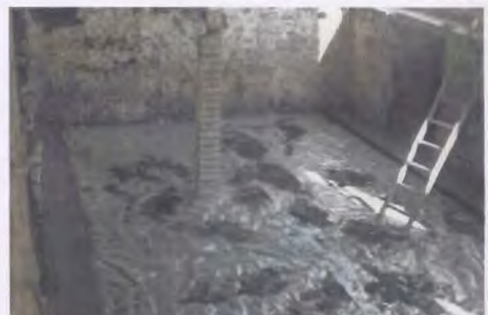
Two views showing the reconstructed upper floor supports and the start of the concrete base to the basement.
