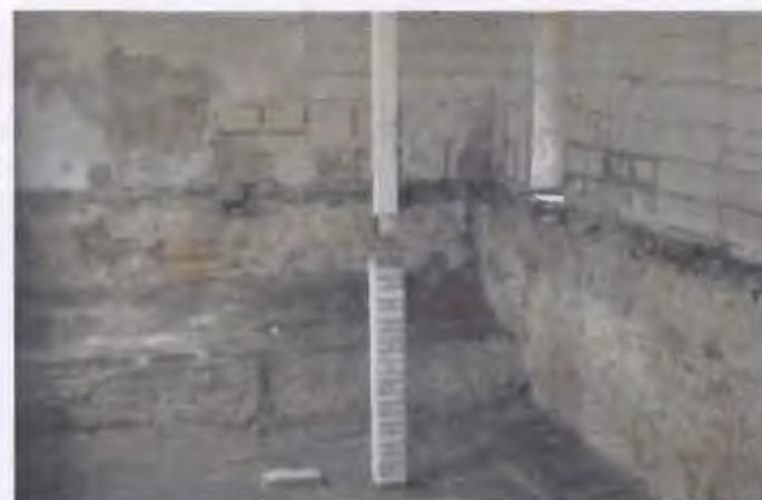
Two views showing the reconstructed upper floor supports and the start of the concrete base to the basement.
