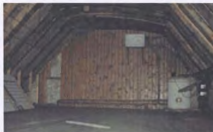
The loft, which had previously been the second floor, showing the pitched pine lining.
