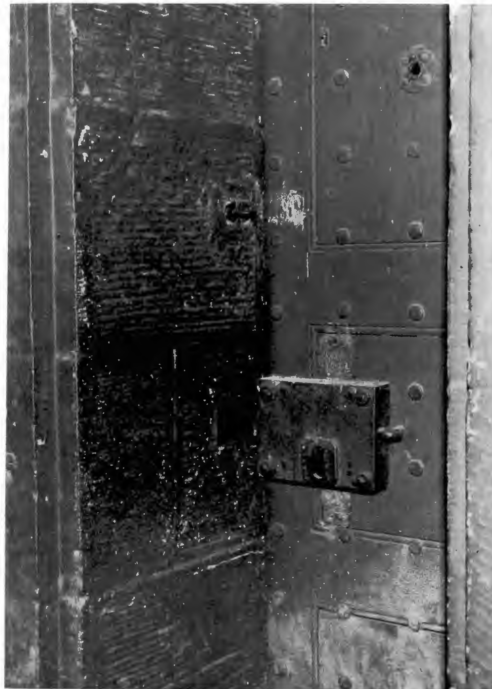
Cell door. Note massive locks, stonework, and Judas hole through which prisoners were observed
