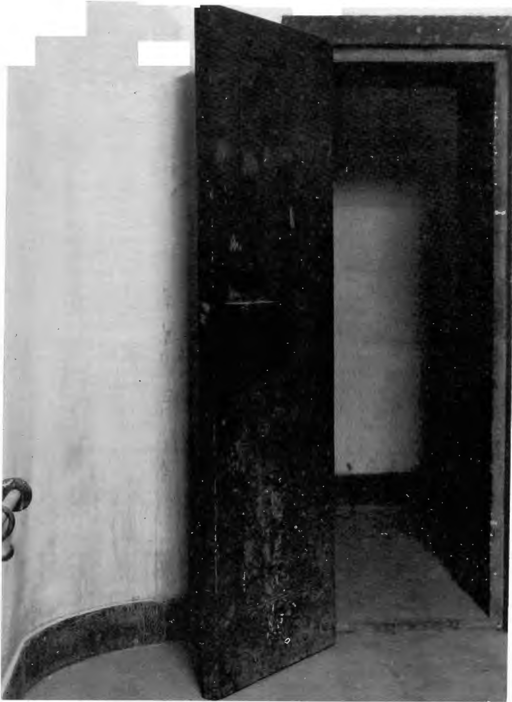
Cell interior to show hammock hooks embedded in cell wall
