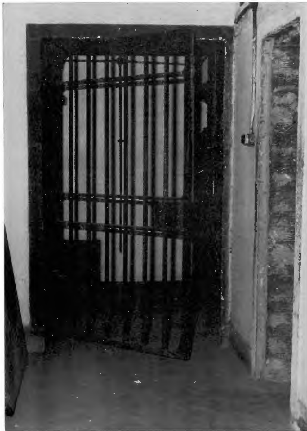
One of the massive steel grilles which cut off one floor from another
