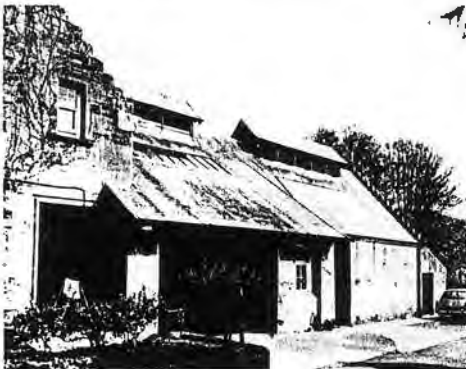
The Garage Block.
