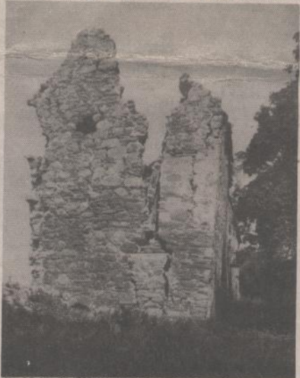
How the manor house has deteriorated over the years. Buildings Trust, was described as "an enthusiastic amateur antiquarian" by George Hume in his BBC Scotland Radio
