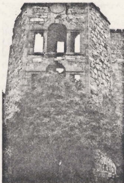
The clock tower of the Spinningdale Mill. The circle above the arched window is the clock which didn't show the time of day but the hours the mill machinery ran during any given day.
