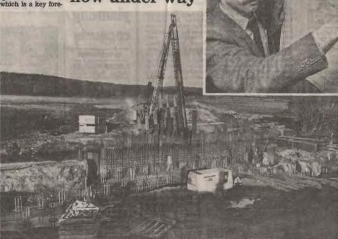
The route leaves the present A9 north of Clashmore and carves its way through a belt of pine trees. The north embankment approach ramp to the Domoch Bridge is being created by Millers out of no less than 100,000 cubic metres
