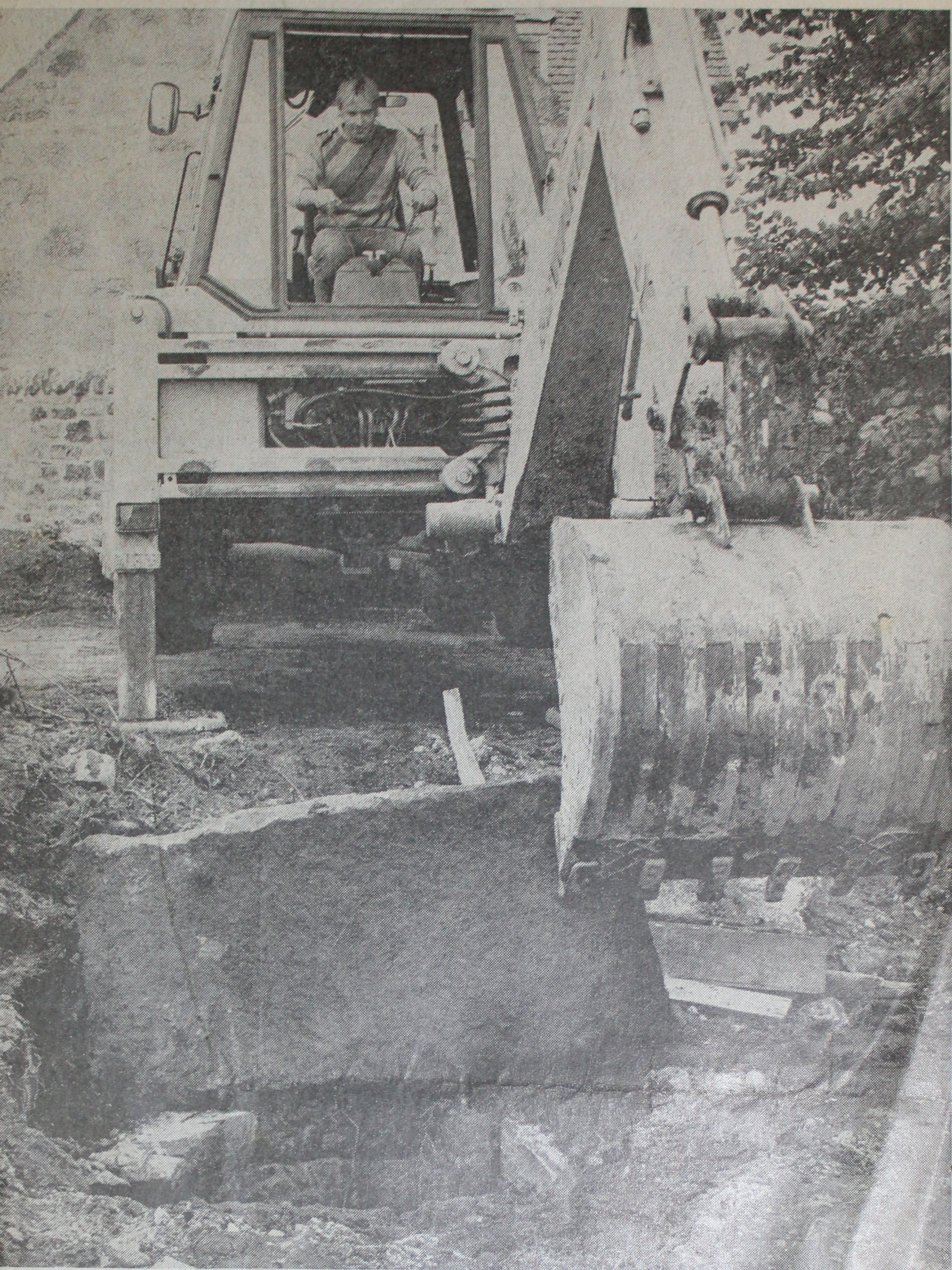
Excavator driver Fraser MacIennan of Rearquhar uncovers what may be the Old Manse Well in Dornoch's Meadows Road. Dornoch Heritage Society are grateful to him, fellow driver Gary Maclean and all Edward Mackay's men for their consideration in the search.
