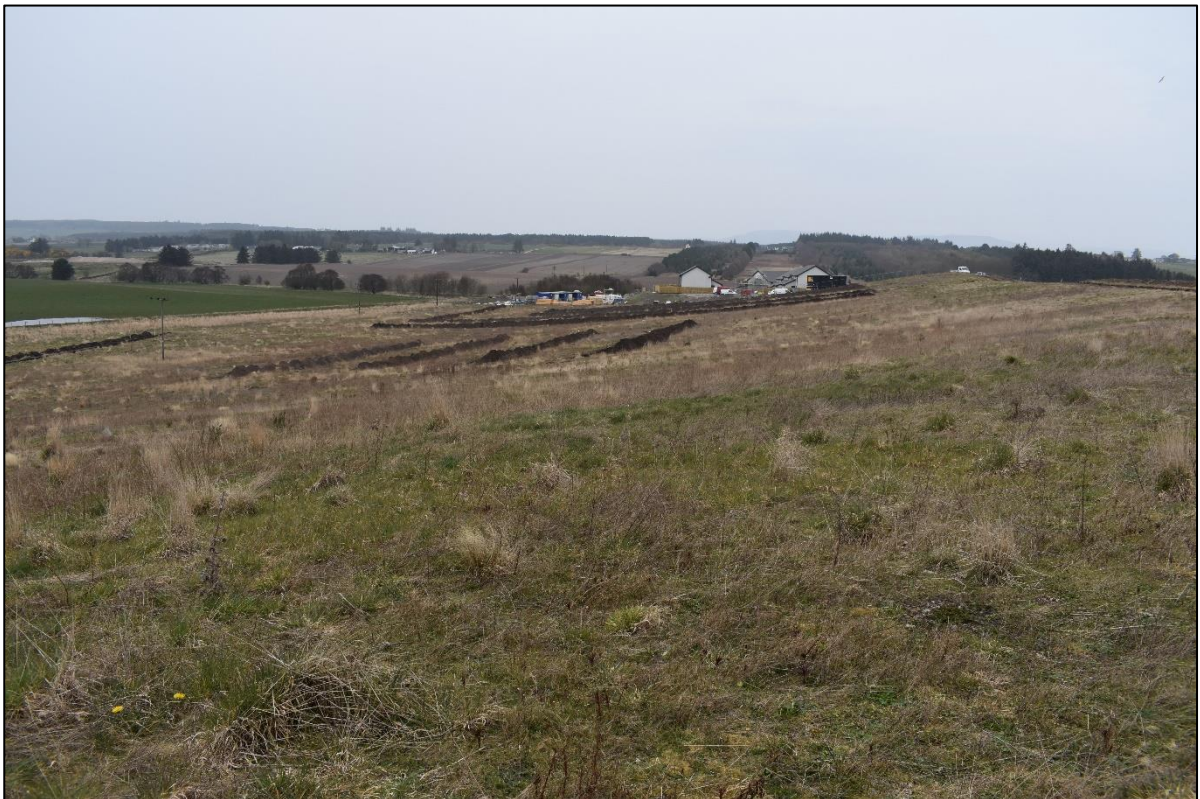
Plate 2: Trenching in progress across the development site
