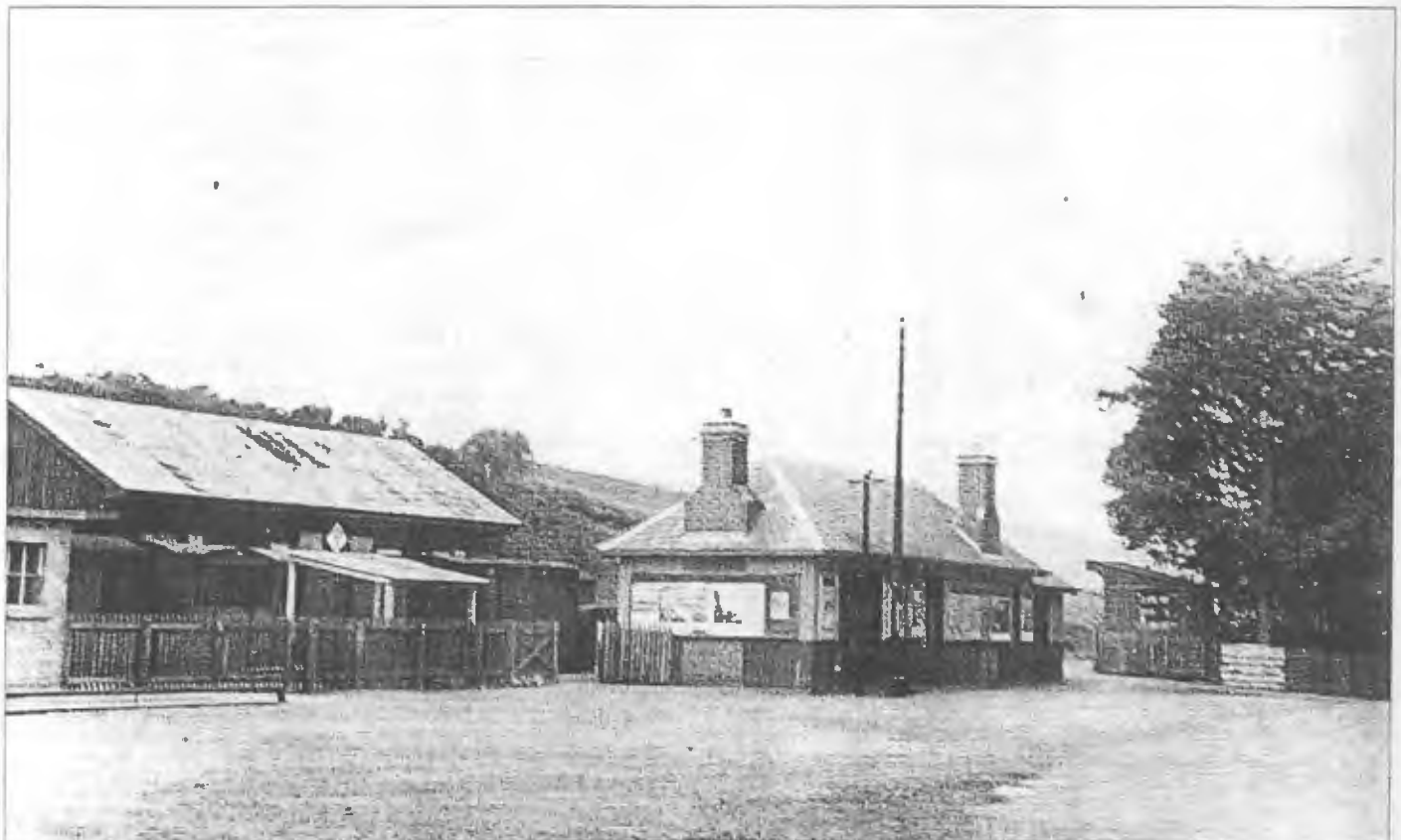
The exterior of Dornoch station, 30 July 1952. When the station opened in 1902 it had a bookshop run by a Mr.Gillespie. The station building was described as having a 'piend' roof - this is an old Scottish word for hipped. The building itself is now preserved. PHOTOGRAPH: F.W.SHUTTLEWORTH
