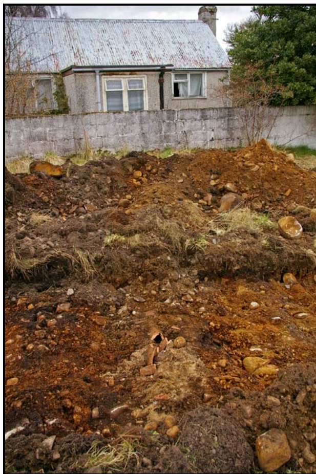
Figure 18 Drain to soakaway, encountered in Trench 1
