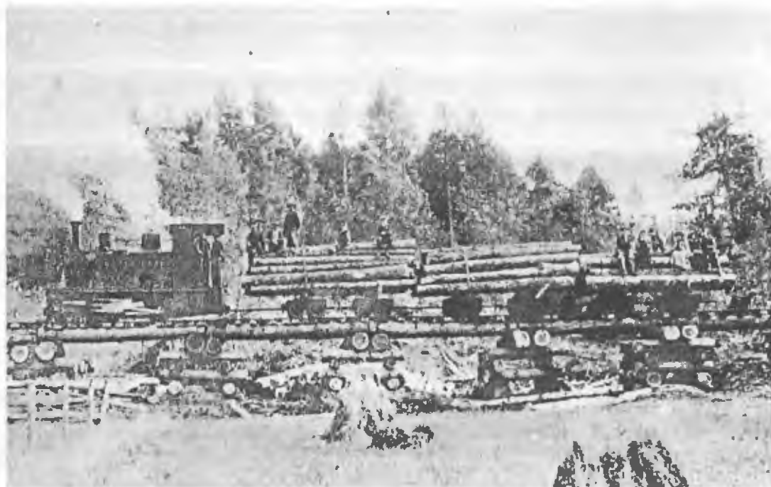
A view of a light railway constructed by 122nd Company of the CFC at Forres, near Elgin in Scotland. The locomotive is a Barclay 0-4-0T 1249 of 1911, which after leaving Forres spent the rest of its life on reservoir construction work. (Authors' collection)
